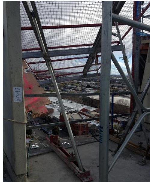
Figure 2. Screen stabilized by push-pull props
