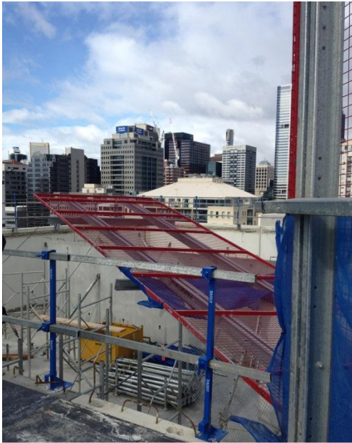
Figure 1. Dislodged Screen
