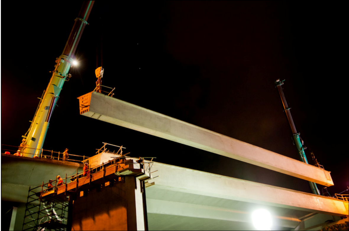
The erection of one of the 100 tonne 45 metre long beams.
