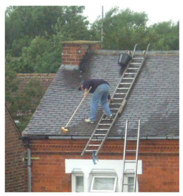
Here we see a couple of likely lads doing a spot of roof cleaning. Clearly their approach to safe ladder set-up and general fall prevention could do with some cleaning up too.
